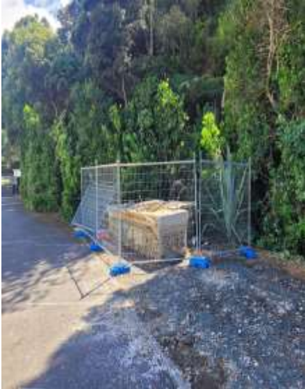
Left: remaining used pontoons to be taken away
